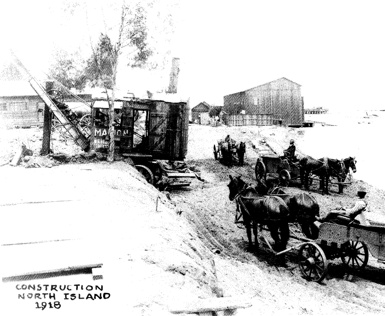
Figure 9. View of shoreline bluffs typical of those found facing San Diego Bay along North Island and Coronado. This photo, taken at the northeast corner of North Island looking north in 1918, shows the bluffs being graded (and the sediment hauled away by carriages) for the construction of seaplane hangars. Spanish Bight is the waterway to the right. Source: Sudsbury 1992.
